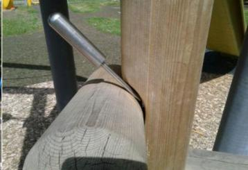
**Finding:** There is/are finger entrapment/s in the ladder climb **Action:** Monitor - No remedial work recommended and the item fails to meet the requirements of BS EN 1176
