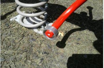
Finding: The end of handgrips and/or footrests have a cross Action: Provide foot grip rests section of less than 15cm2 and fail to meet the requirements of BS EN 1176 Part 6
