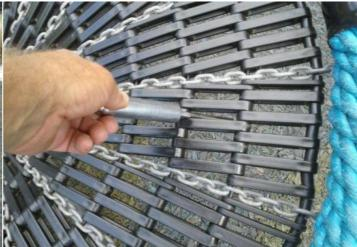
Finding: There is/are finger entrapment/s in the basket and Action: Monitor - No remedial work recommended the item fails to meet the requirements of BS EN 1176 Part 1
