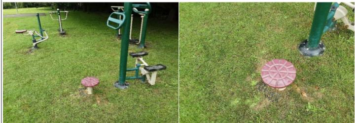
Finding: The rotating user station is not appropriately marked with a guideline of user direction and/or the original position as required by BS EN 16630
