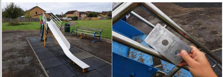
Finding: The item fails to meet the requirements of BS EN Action: Monitor - No remedial work recommended 1176 Part 1 4.2.7.2 head and neck entrapment in the barriers and/or steps
