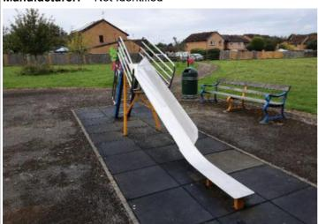
Finding: The surfacing dimensions are significantly short and do not meet with the requirements of the current applicable standard (1500mm required / 700mm provided) Risk Level: Surface:
