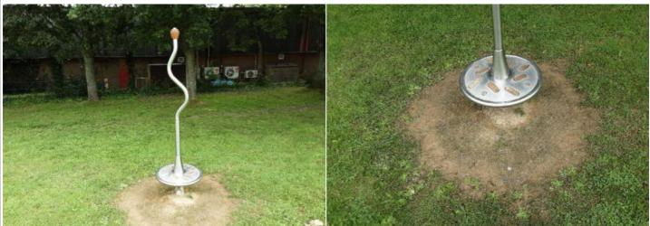
Finding: The grass mats are silted up and the soil is compacted; this may have an effect on the impact absorbing ensure the correct surface qualities are maintained for the properties of the surface
