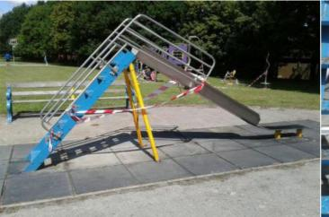
**Finding:** The surfacing dimensions are significantly short and do not meet with the requirements of the current applicable standard (1500mm required / 700mm provided)
