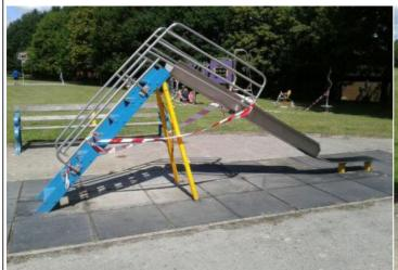
**Finding:** The height of the barrier(s) is insufficient and fails **Action:** Monitor - No remedial work recommended to meet the recommendations of BS EN 1176 Part 1
